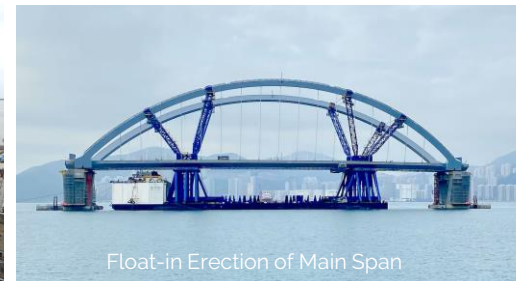
Marine Transportation of Main Span
