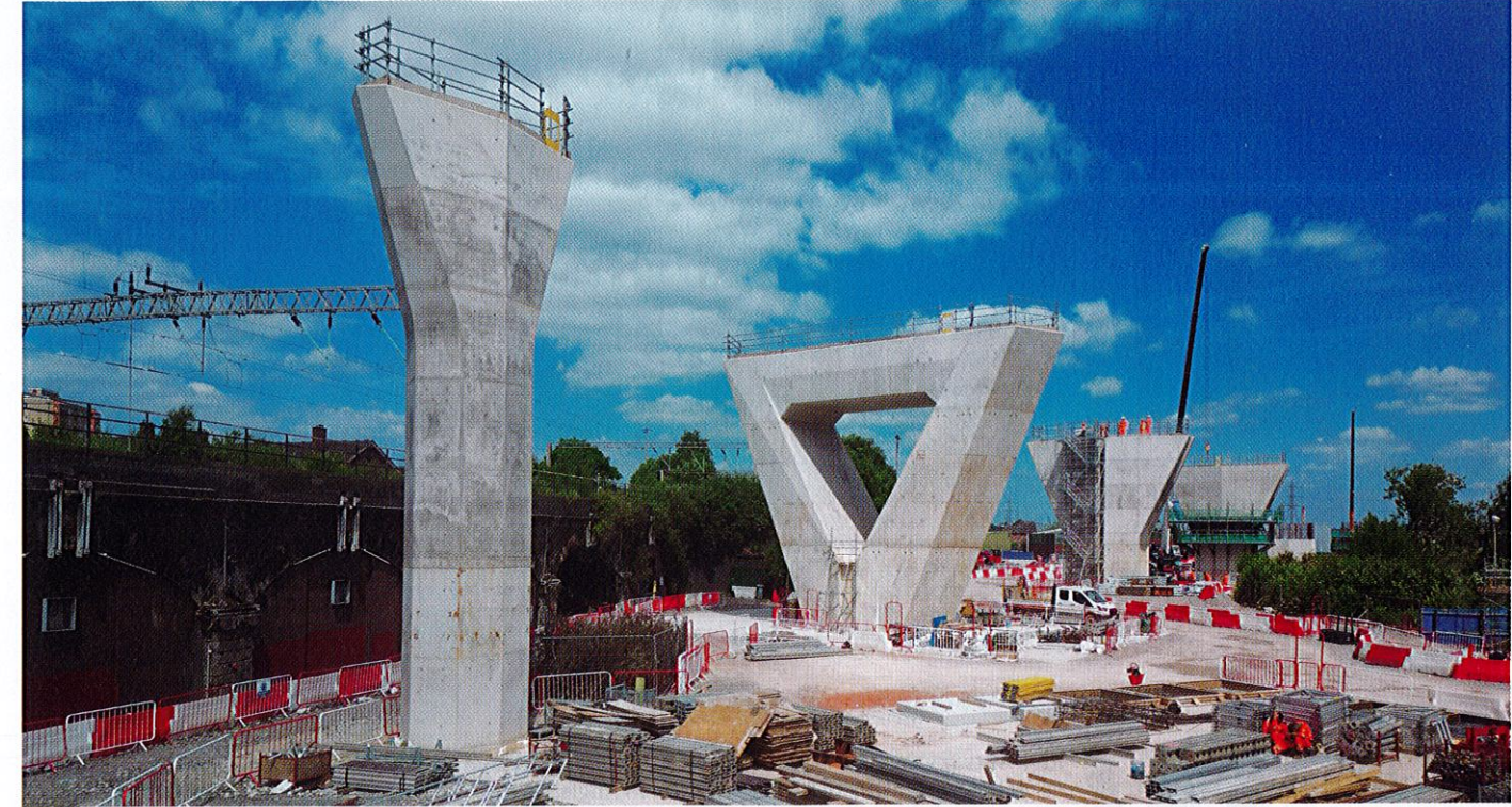
The four huge piers for Curzon 2 in Birmingham reflect both the needs of the bridge in its permanent state, and the stresses that the piers experience during one of the longest bridge launches ever undertaken in the UK. (Photo credit: HS2 Ltd)
