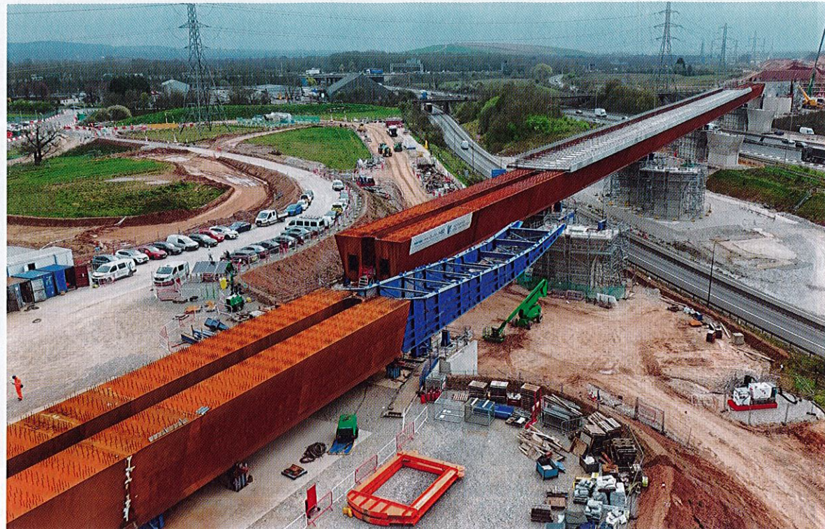
A 45-strong crew were assembled to carry out the slide and subsequent checks on a 107m section of the west deck over an M6 slip road, with the slip road being scheduled for closure for less than 48 hours. (Photo credit: HS2 Ltd)
